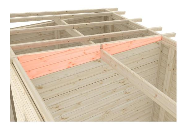
**8. DIAGONAL SUPPORTS** Before you start fixing the roof board, make sure that the walls of the cabin are straight. The delivery includes separately installed diagonal supports, it is recommended to install them at this stage.
