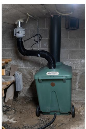
Place the composting unit with the open lid below the waste pipe.
