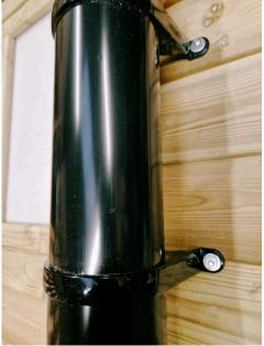
Fit the two support brackets on the pre-formed vent pipe. From the outside, offer the support brackets up to the protruding bolts and loosely secure with a washer and nut. It can be helpful to have someone inside the cabin to keep the bolts in place until the washer and nut is on.
