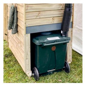
Attach the short flexible 110mm vent pipe connector to the outlet on the top of the WooWoo GT composting toilet lid and check that the other end is in a good position to connect onto the bottom of the flue.
