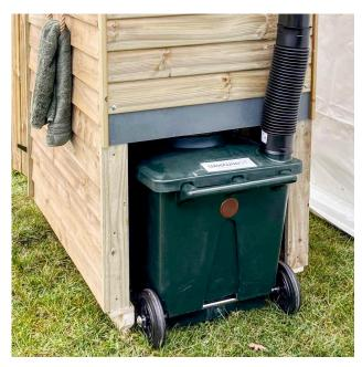
Finally, attach the leachate pipe to the outlet on the rear of the composting container and run this to your soak-away pit or leachate container.
