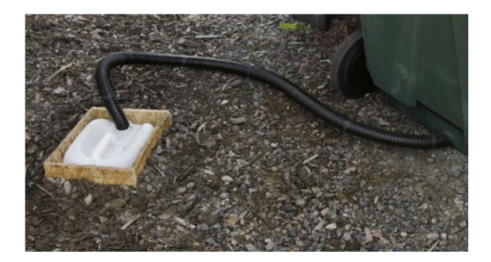
In public sites where the overall use is higher, we'd recommend installing a urinal as well. This will help to handle possible peaks in the use and reduce the amount of leachate. From urinals, the urine can be led back to the ground through a soak-away pit. Alternatively, the urine can be collected directly to a container after which it can be used as a fertiliser, or disposed of in a suitable manner.
